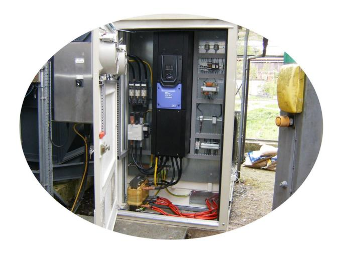
(VSD) control system. Motor Control Warehouse in conjunction with BRE, have now designed, built and installed a fully automated VSD control system using three Invertek Optidrive HVAC, 160kW, IP55 AC Drives. The drives are housed in purpose built glass fibre weather resistant enclosures.
